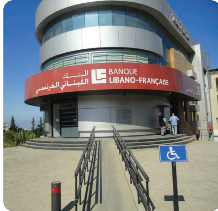
Hazmieh branch equipped with a ramp.
